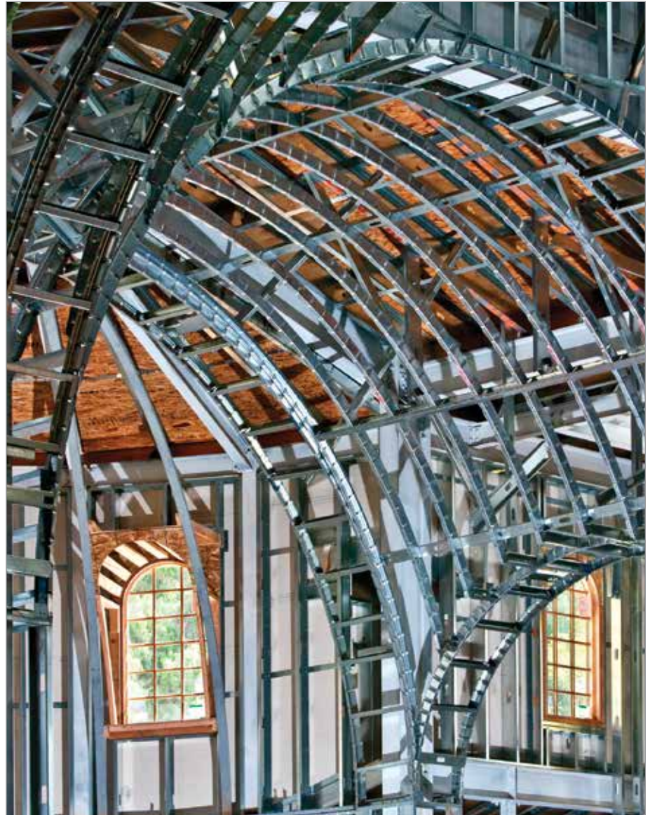
Complex Surface and Interior Dome St. Andrews Orthodox Christian Church / Riverside, CA
