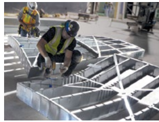
Unitized Panels - Space Shuttle Atlantis Attraction, Kennedy Space Center, FL
