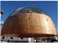
Forming this lofty dome with a light weight Curved-Right® Dome Formwork assembly made short, safe, work of the job. The Radius Track Team designed and fabricated cold-formed steel (CFS) framing for the large mosque dome and the 2 bathhouse domes.
