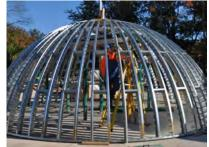
The light weight of the CFS framed dome formwork assembly allowed them to build the 3 forms on the ground and hoist each into place with a crane. The concrete subcontractor estimated this saved almost one month of schedule.
