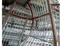
Visually interesting, the mass of each curved surface isolates each space acoustically. Curved-Right® framing elements help support 3" shot crete, 1 layer of varnished MDF, and 2 layers of gypsum wall board.
