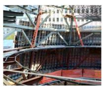
Unitized CFS panels, single sourced by Radius Track® from sub-frame up to finished surface, were used to cost effectively construct this complex feature in the tight urban site.
