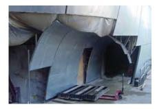
The walls of the hull were curved in both vertical and horizontal dimensions. Curved-Right® studs were pre-curved to the exact radius specified.
