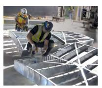
Radius Track® fabricated unitized CFS framing for the theater's arches using design data extracted from their 3D model used for clash detection and fit.
