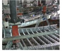
Radius Track's 3D model provided the data for them to fabricate 3,432 curved studs, 2,632 curved track framing pieces, 94% one of a kind. Curved box beams set in place using laser technology connected Acoustic Sails framed in curved track and studs to stalactites via 3-axis adjustable hanger assemblies.
