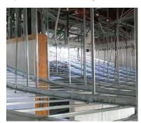
A Curved-Right® pre-curved framing solution allowed J&J Acoustics to frame 99% of the ceiling using scissor lifts instead of full scaffolding.
