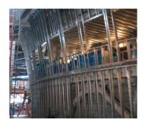
Curved-Right® pre-curved stud, track, and header elements frame the compound curves for the sculptural wall and support the GFRG panel assembly.
